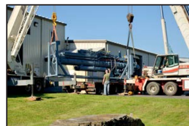
Each of the 51,000 lb. cylinder assemblies required a custom stand for assembly and transportation.
