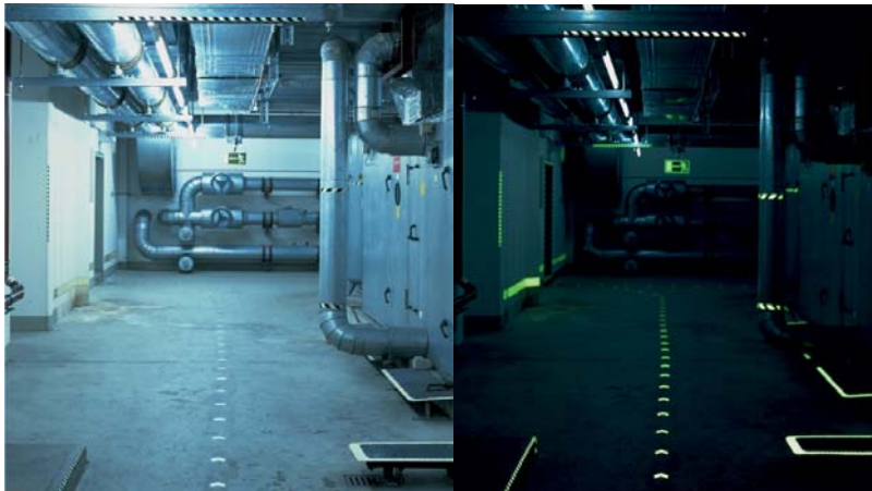
Utility Bunker with obstacles and exit path marked.
