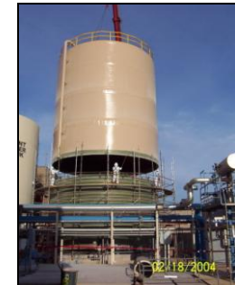
350,000 gallon potable water tank
