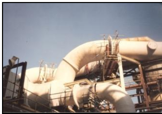
FRP duct fabrication & field installation
