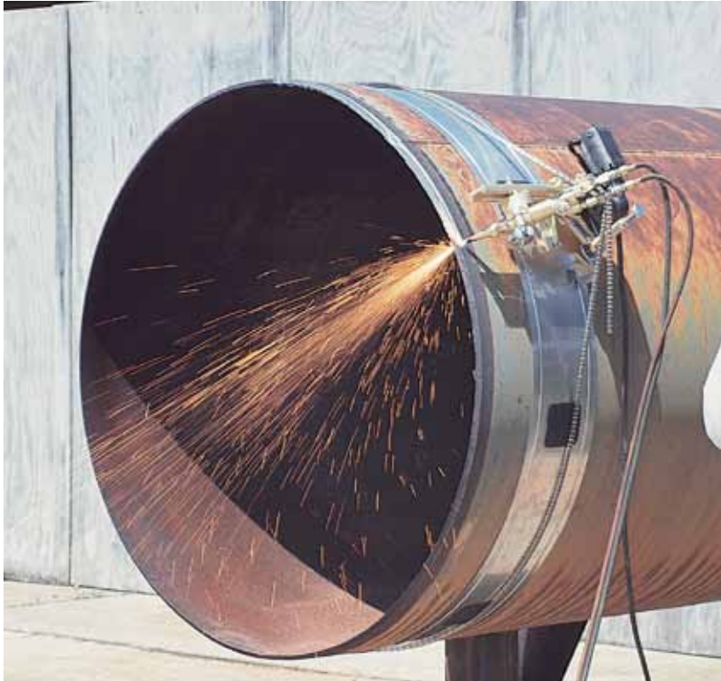
Cutting 48" pipe with Band-Type Pipe Beveler
