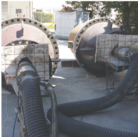
Multiple pieces ready for cure simultaneously often provide cost savings.
