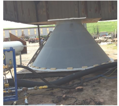
Refractory cure on Transition Cone.
