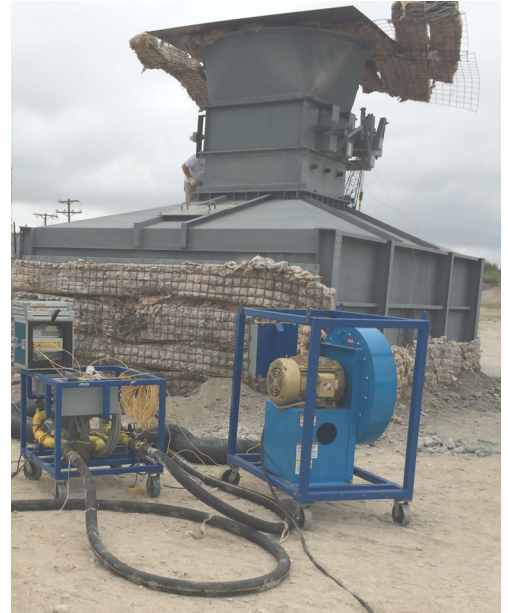
Refractory cure on Convection Box with Exhaust Stack Transition and Baffle System.
