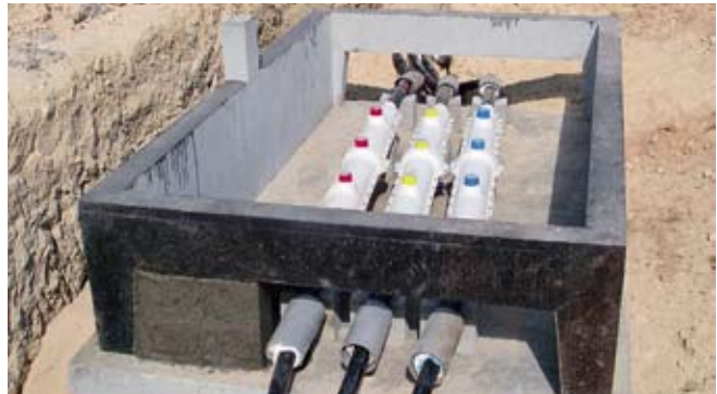
Joints with polyester protection box in a concrete pit
