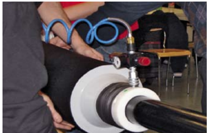
Assembling-friendly installation of a slip-on joint by "air cushion" method
