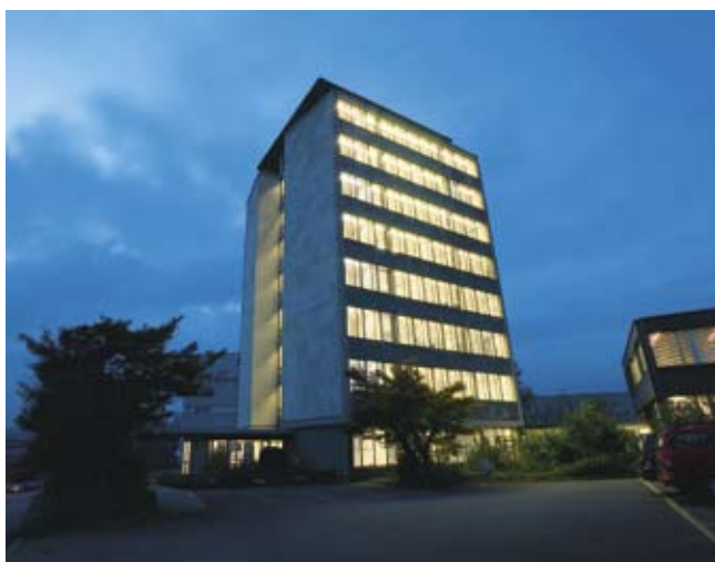
Headquarters of Brugg Cables
