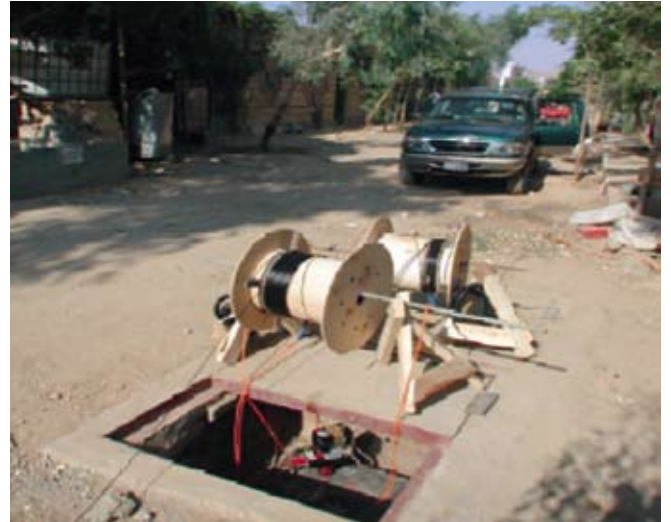
PD measurement on customer in Egypt
