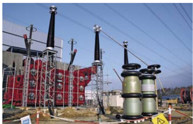
Commissioning test on-site at 420 kV porcelain terminations in Germany
