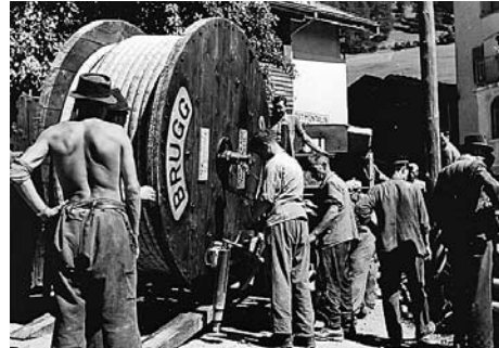
Laying of 420 kV oil-filled cables in Switzerland in the 1960s
