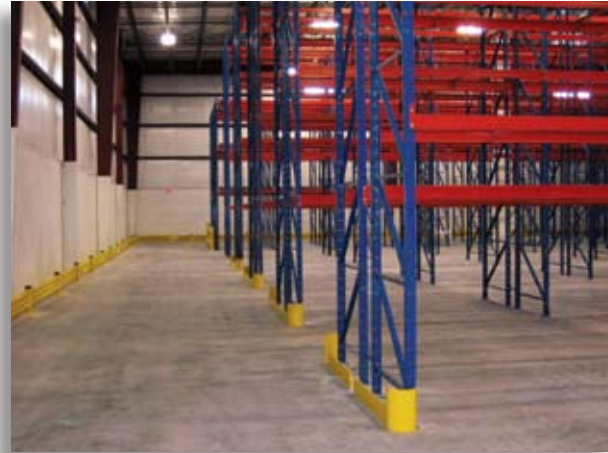
Wall and rack protection
