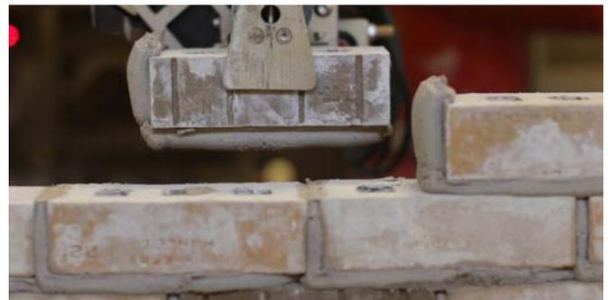
**Construction Robotics' flagship product is the Semi-Automated Mason (SAM), a robotic bricklaying system. This automated machine helps masons improve efficiency.**
