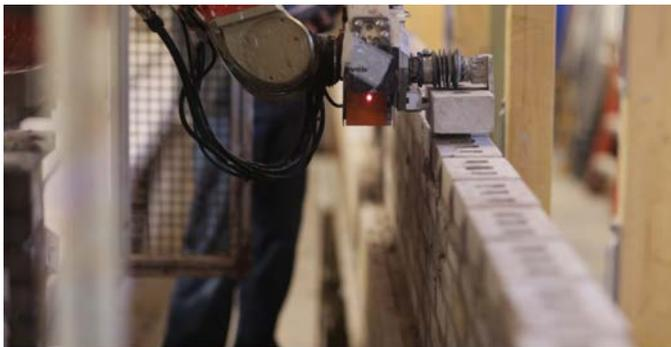
**SAM's laser system measures each brick individually and can detect even small variances between the bricks.**
