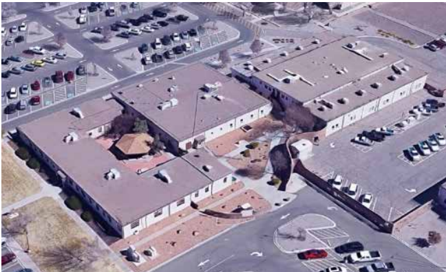
The development and deployment of a DC microgrid serving Kirtland AFB Civil Engineering facilities will provide an immediate resiliency benefit, while serving as a test bed that evaluates technology benefits across the DoD.
