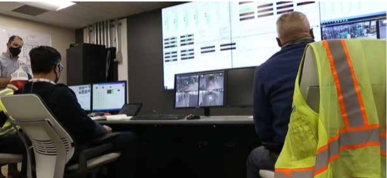
Marine Corps FRCS personnel are shown monitoring MCAS Miramar's microgrid for potential energy savings, electrical anomalies, and malicious activity. U.S. Marine Corps image
