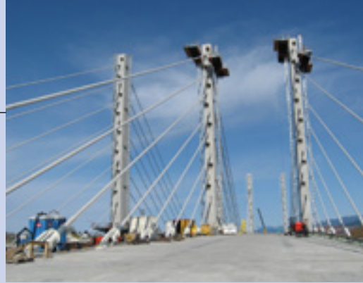
Gajo Arch Bridge, Geoje City, South Korea 80 DYNA Grip® Stay Cables Maximum cable length: 31 m Cable size: DG-P12
