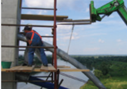
Saddle Pipe Installation
