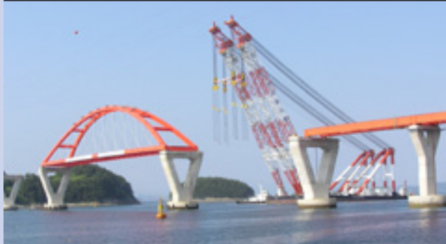
Gajo Arch Bridge, Geoje City, South Korea 80 DYNA Grip® Stay Cables Maximum cable length: 31 m Cable size: DG-P12
