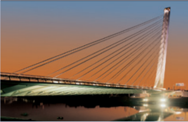
Alamillo Bridge, Sevilla, Spain 28 DYNA Bond® Stay Cables Maximum cable length: 292 m Cable size: DB-E61
