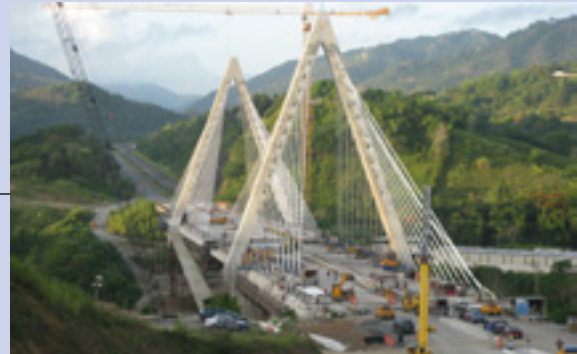
Ziegelgraben Bridge, Germany 32 DYNA Grip® Stay Cables Maximum cable length: 176 m Cable size: DG-P37
