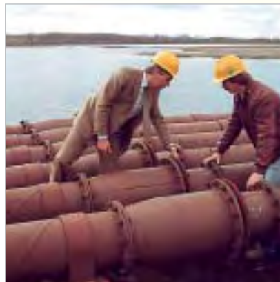
Expansion joints in a hydraulic bottom ash pipeline.
