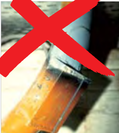
Simple but not very efficient: Welded patches on steel pipes.
