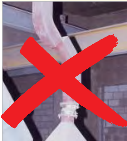
Concrete filled wear boxes are a short term solution.
