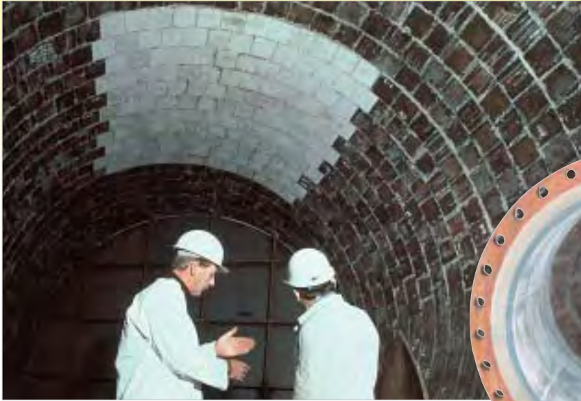
ABRESIST and KALCOR combination within a dust collection system in a steel plant. The raw gasses in the duct have a temperature of 250 °C / 482 °F and are loaded with sinter dust. The impact area opposite the gas inlet is lined with KALCOR.
