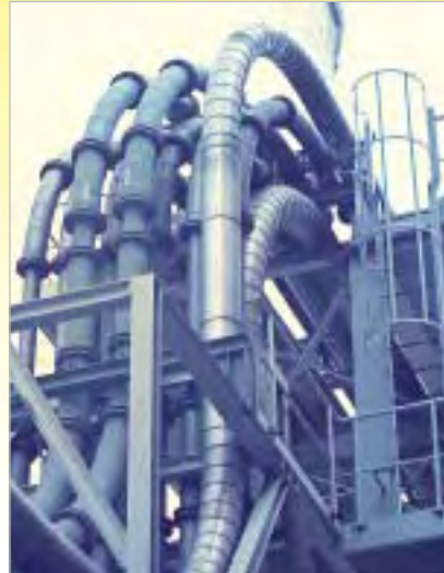
Fly ash pipelines in a coal fired power station.
