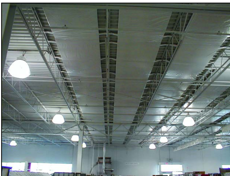
Kinetics Model S4 Panel Absorber mounted in the overhead trusses control unwanted reverberant noise to acceptable levels.
