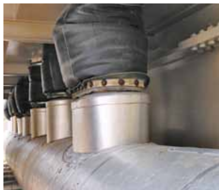
KE ® Fabric Expansion Joints installed in a Pipe Penetration System.
