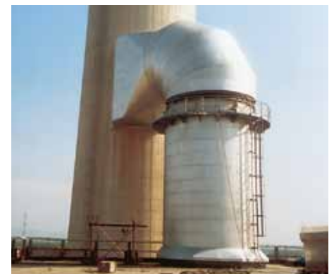
Expansion Joint for Chimney Connections.
