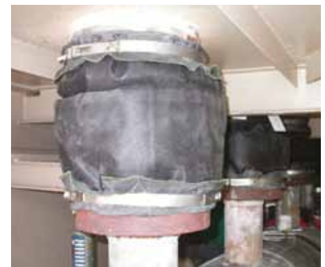
Pipe Penetration with external Insulation.
