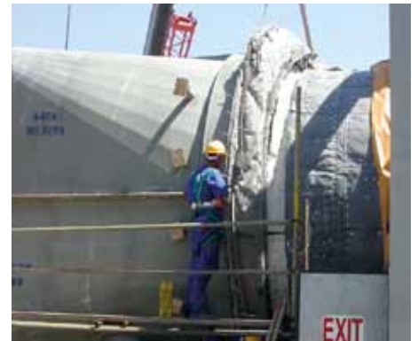
Installation of KE® Fabric Expansion Joint.
