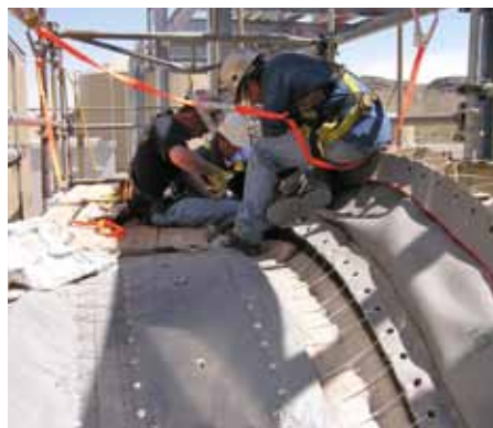
Replacement of KE® Fabric Expansion Joint.
