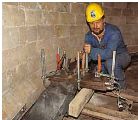
Lining Joint Sealings in Chimneys.
