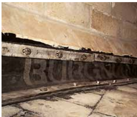
Lining Joint Sealings in Chimneys.
