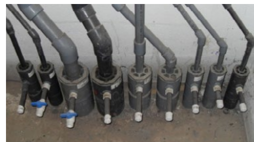
The IPEX Guardian™ Vinyl double containment system was required for underground runs, which transitioned to IPEX single wall PVC and Corzan CPVC inside the facility.
