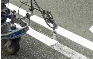
In the *road marking industry*, our hydrocarbon resins are combined into hot-applied thermoplastic road marking materials to ensure pavement markings are durable and visible.
